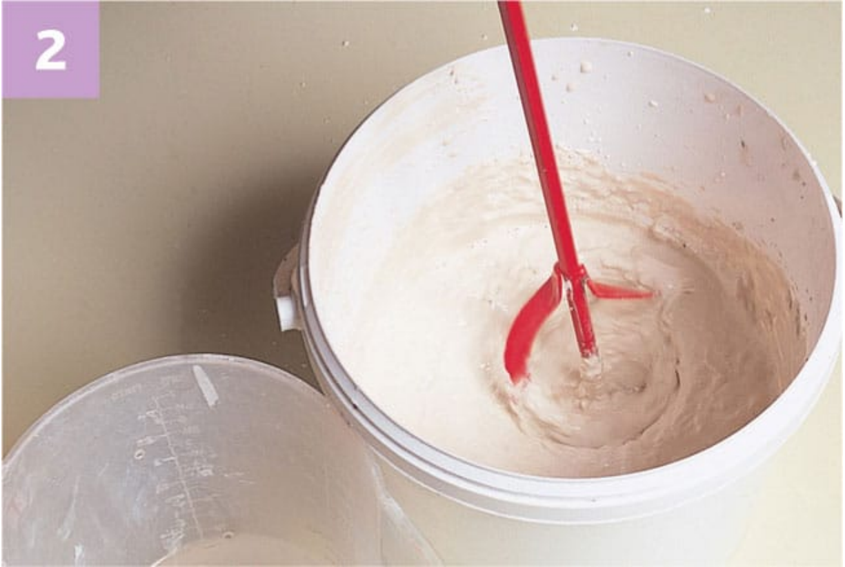
2 Use a metal mixing blade attached to an electric drill to blend the dry powder into the water. The finished consistency should be like thick cream.
