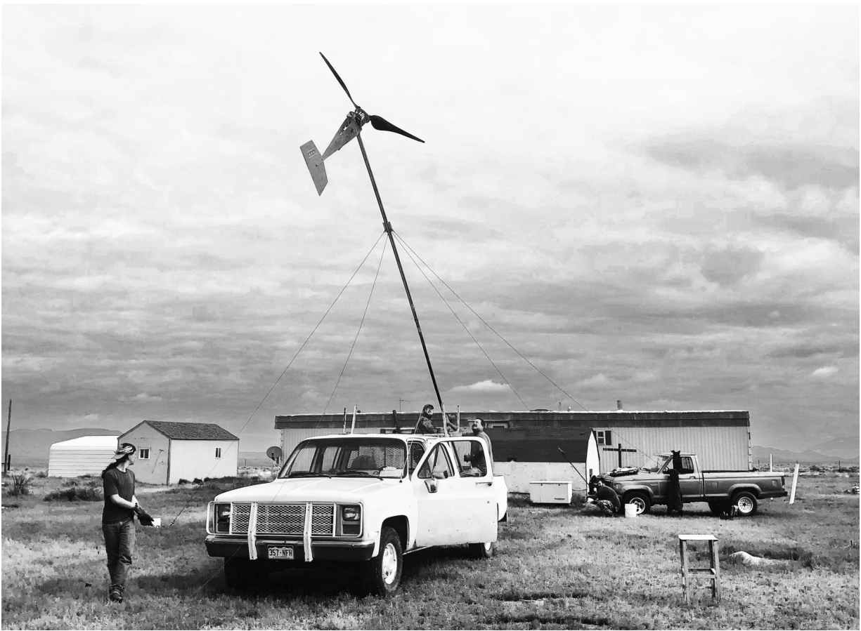
Raising the wind turbine
