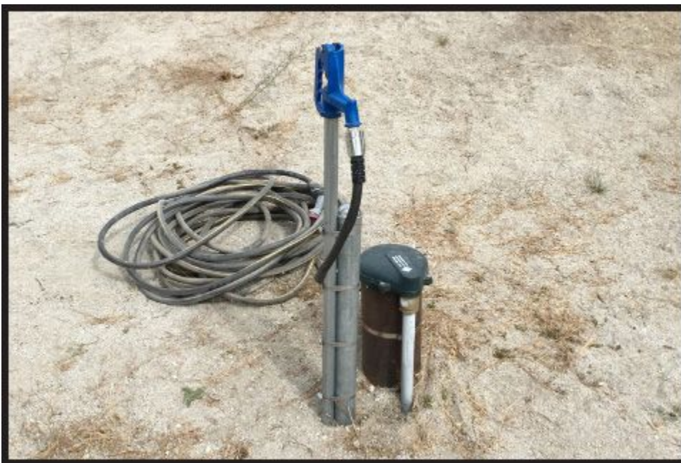
Well pipe and freeze-free spigot
