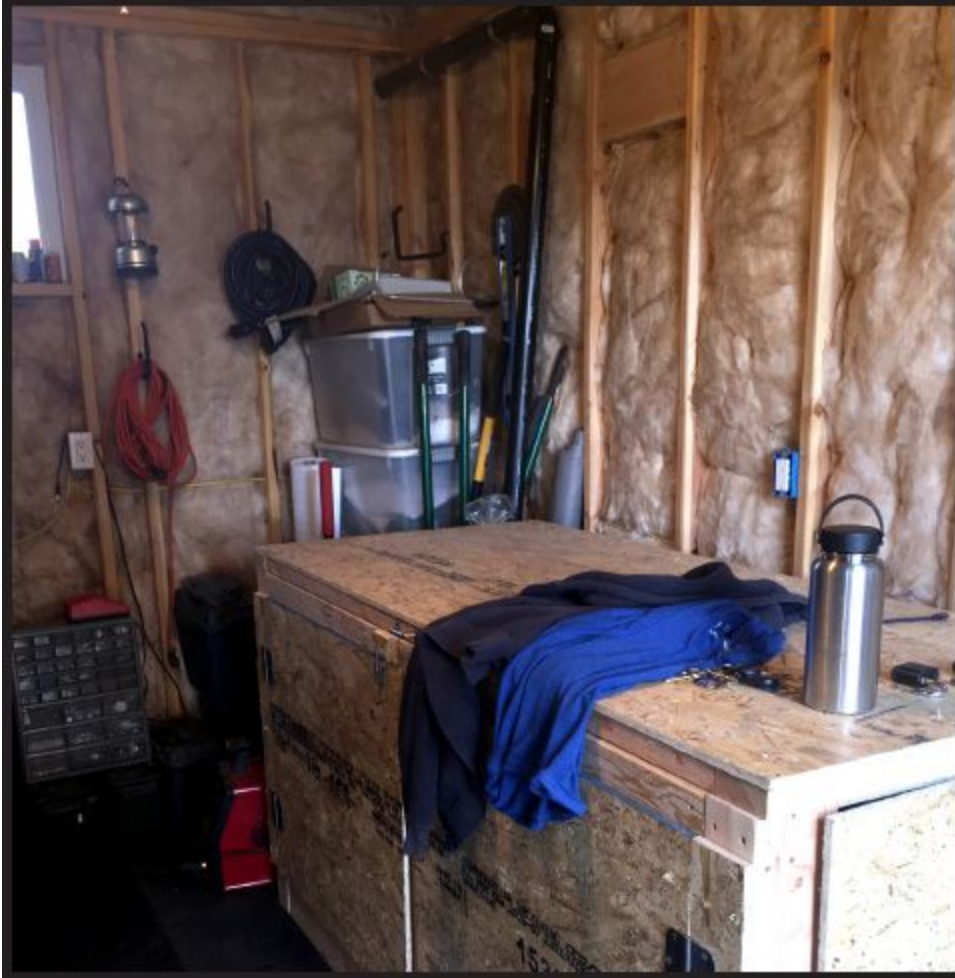
Inside my power shed
