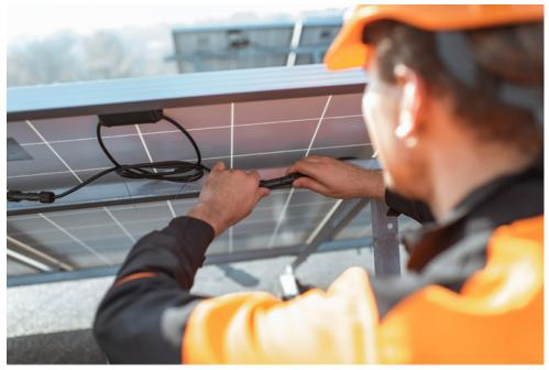
To avoid arcing when the MC4 is disconnected, a breaker should be installed near the connection to open the circuit without the risk of arcing. MC4 connectors are rated for 30 A and are designed for 12 and 10 AWG (4 and 6 mm2) conductor sizes.
