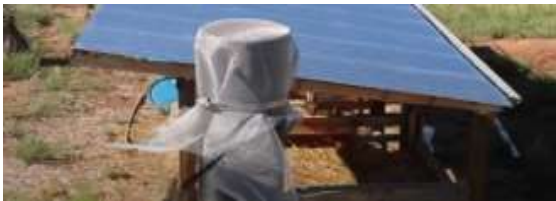
16. Put the vent cap over
