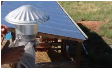
17. Put a couple of screws to hold
