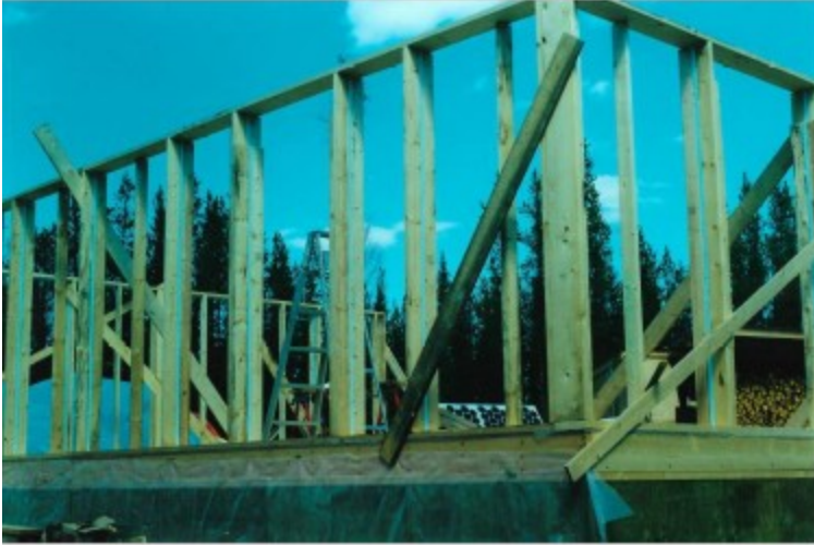
First floor framing
