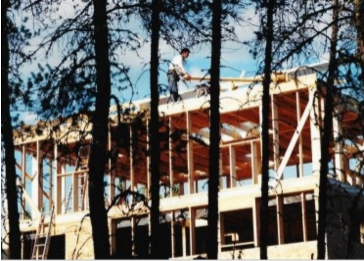
Second story framing
