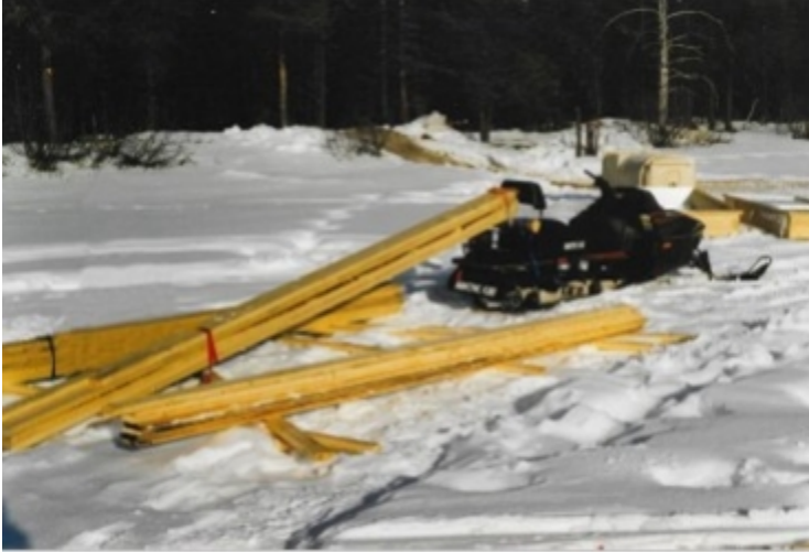
Snowmobile used to move supplies from lake to house site
