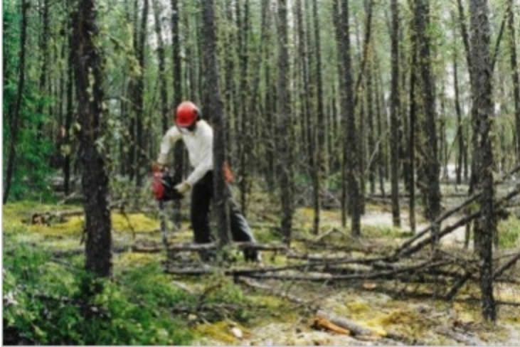
Clearing the land
