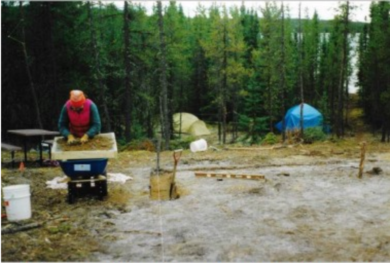
Sifting gravel from the sand for house foundation
