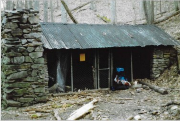
Stone shelter in Smoky Mountain National Park
