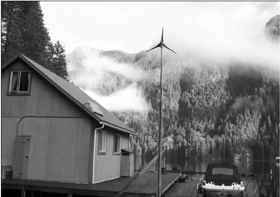
Wind generator at Cabin Number 3
