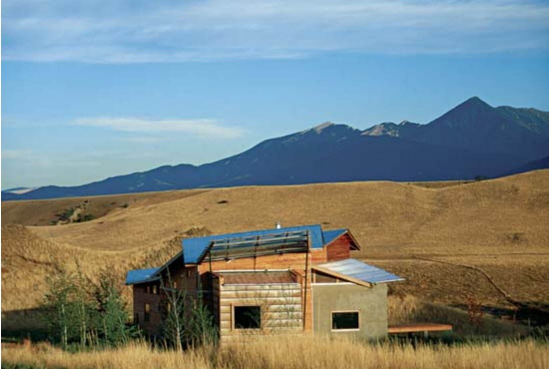
Folds in the roof provide for water collection points. Cisterns located below the roof valleys collect water and snow for watering the indigenous plants.
