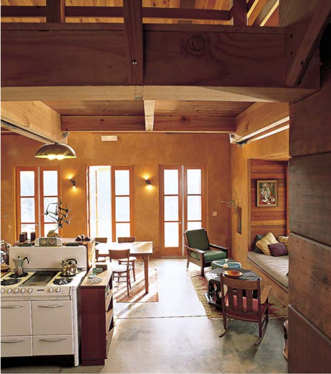
South-facing french doors bring light and solar heat into the house in the winter. The light and heat are blocked in the summer by the porch trellis.
