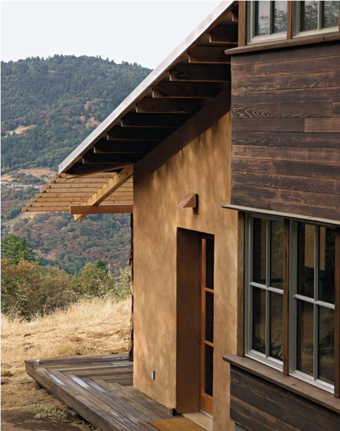
Reclaimed wood is used for exterior siding along with a colored clay finish over the straw bale infill wall system.
