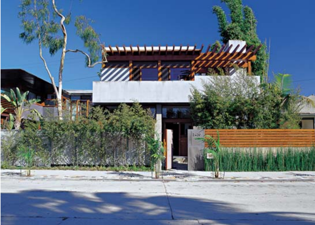
The street-side entry to the house is enclosed with a rammed-earth wall, built from fly ash, decomposed granite sand, and cement. A thin garden space is filled with horsetail reeds and king palms.
