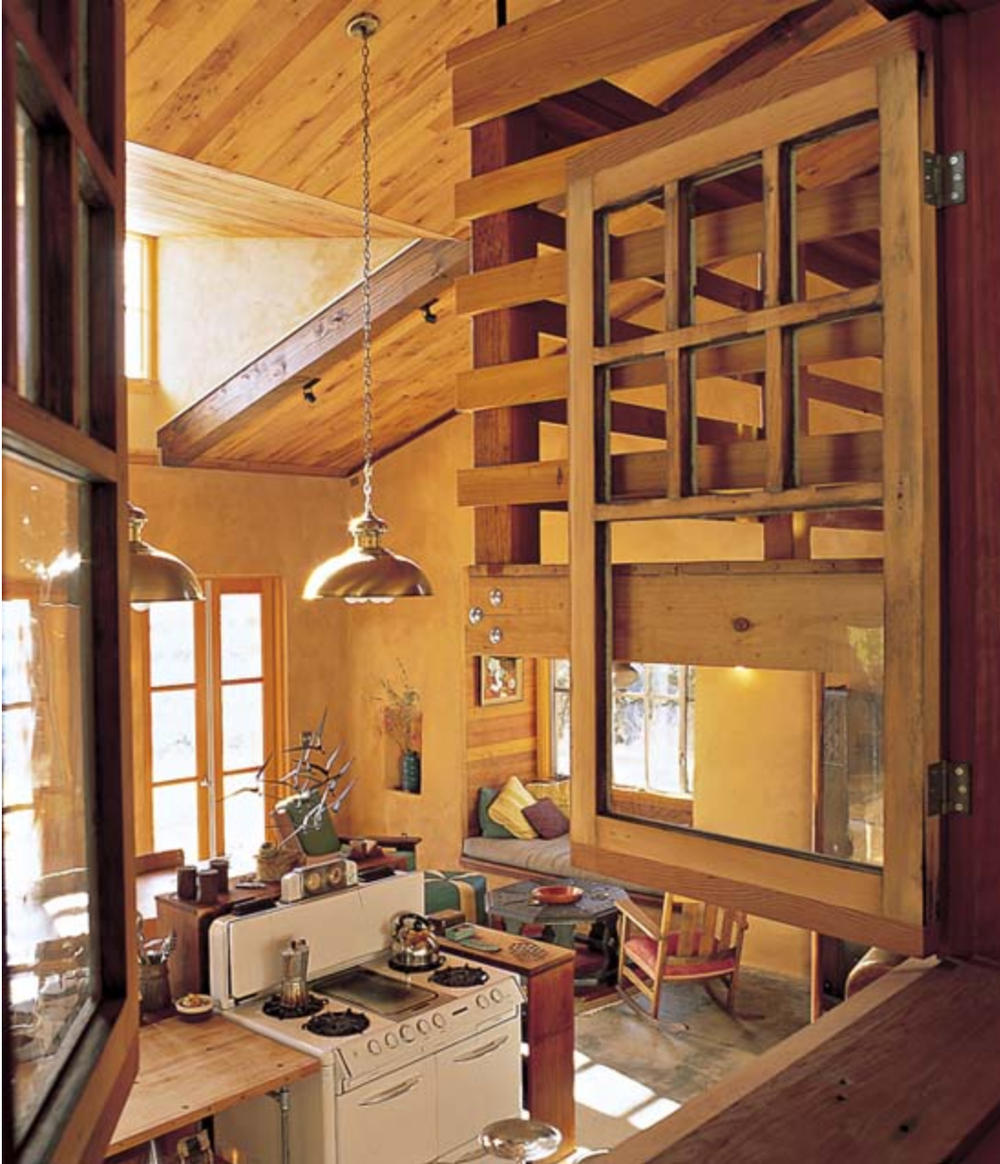
Operable interior windows from the second-floor bedrooms allow the house to ventilate by creating a cross-breeze through the house.
