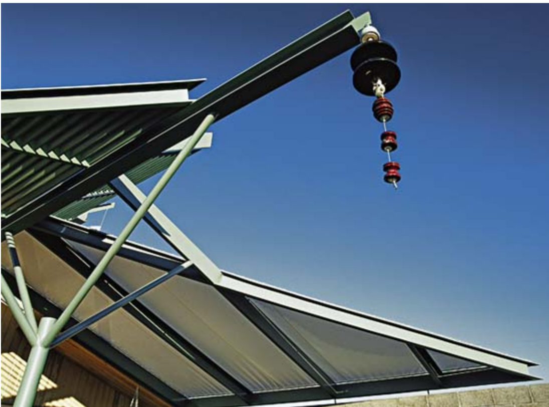
A whimsical rain chain hangs from the end of the scupper, which brings rainwater to the cistern.
