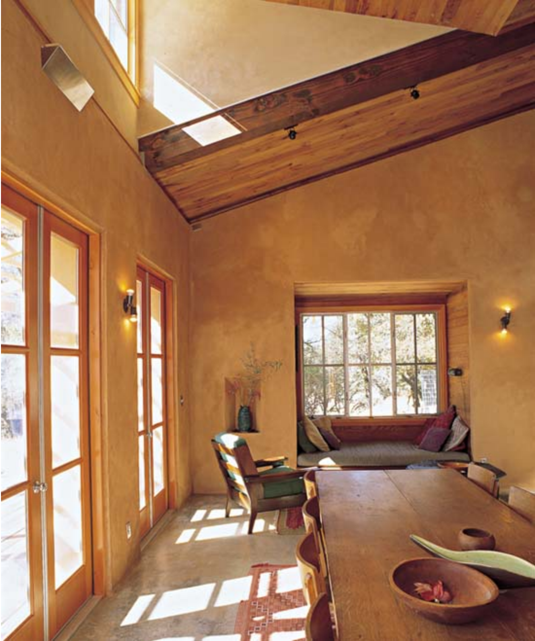
Concrete floors with radiant heat warm the house while highly insulative straw bale walls help to retain the temperature inside.
