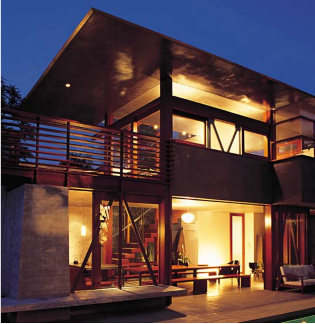
At night the house glows, making apparent the interwoven relationships between inside and out, ground and second floor, including a large balcony off of the children's playroom.
