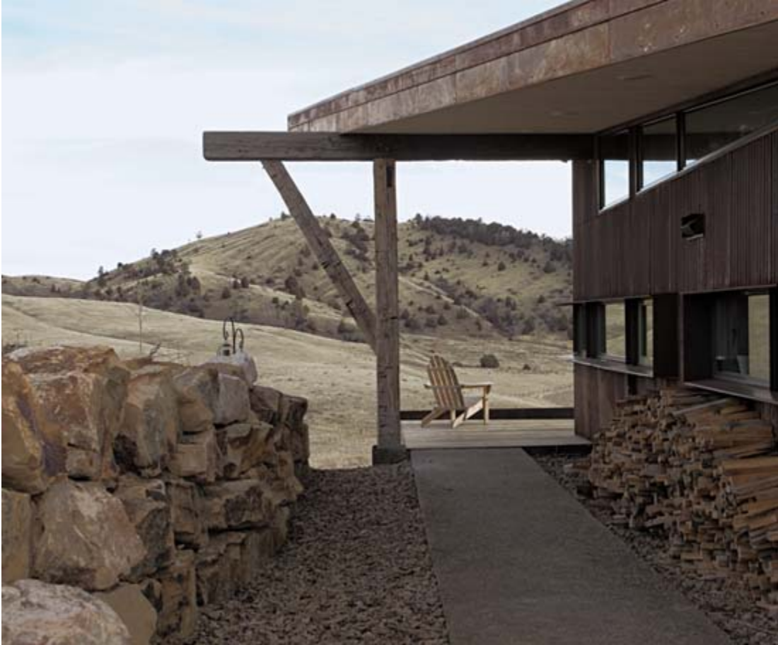
An outdoor breezeway built of reclaimed timbers provides protection from the wind and a passage to the deck space.
