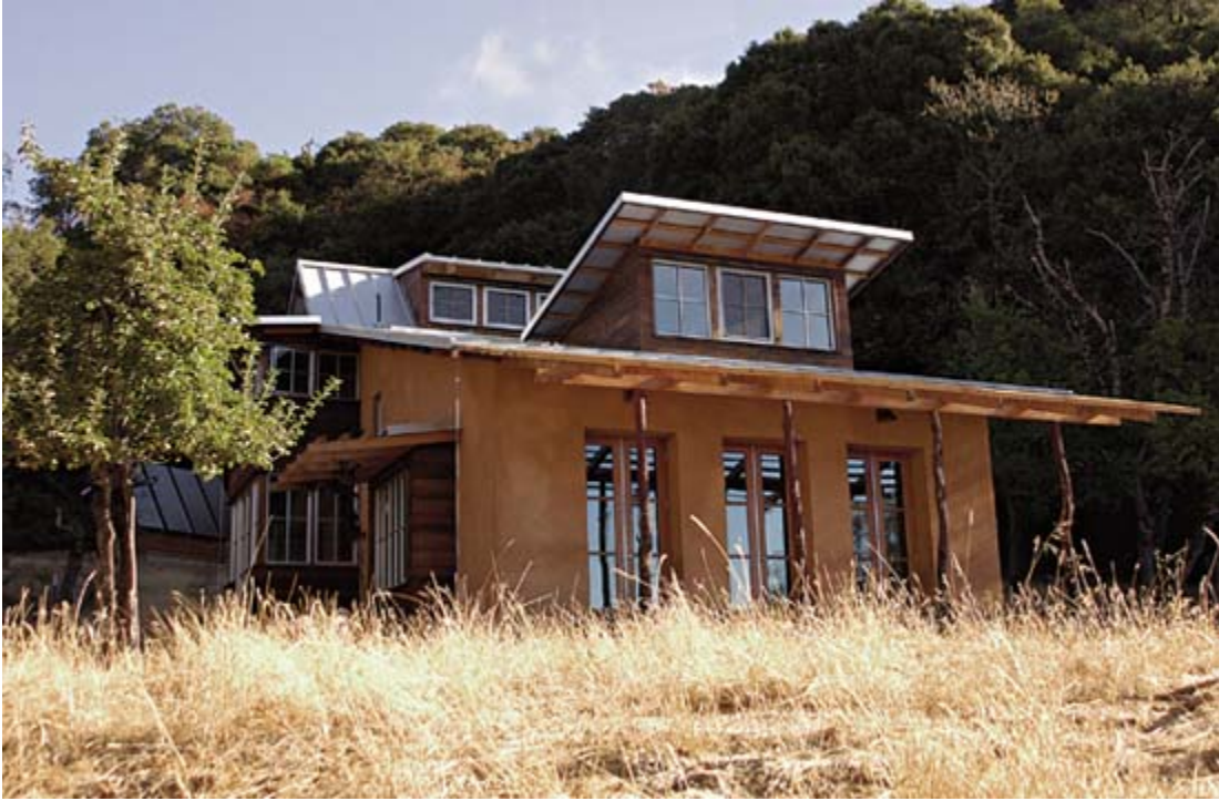
A series of french doors and operable celestory windows work together to naturally ventilate and cool the house.
