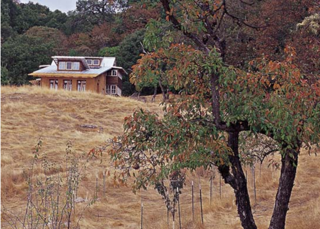
A series of PV panels mounted directly to the roof of the house provide all of the electrical energy requirements for the house.
