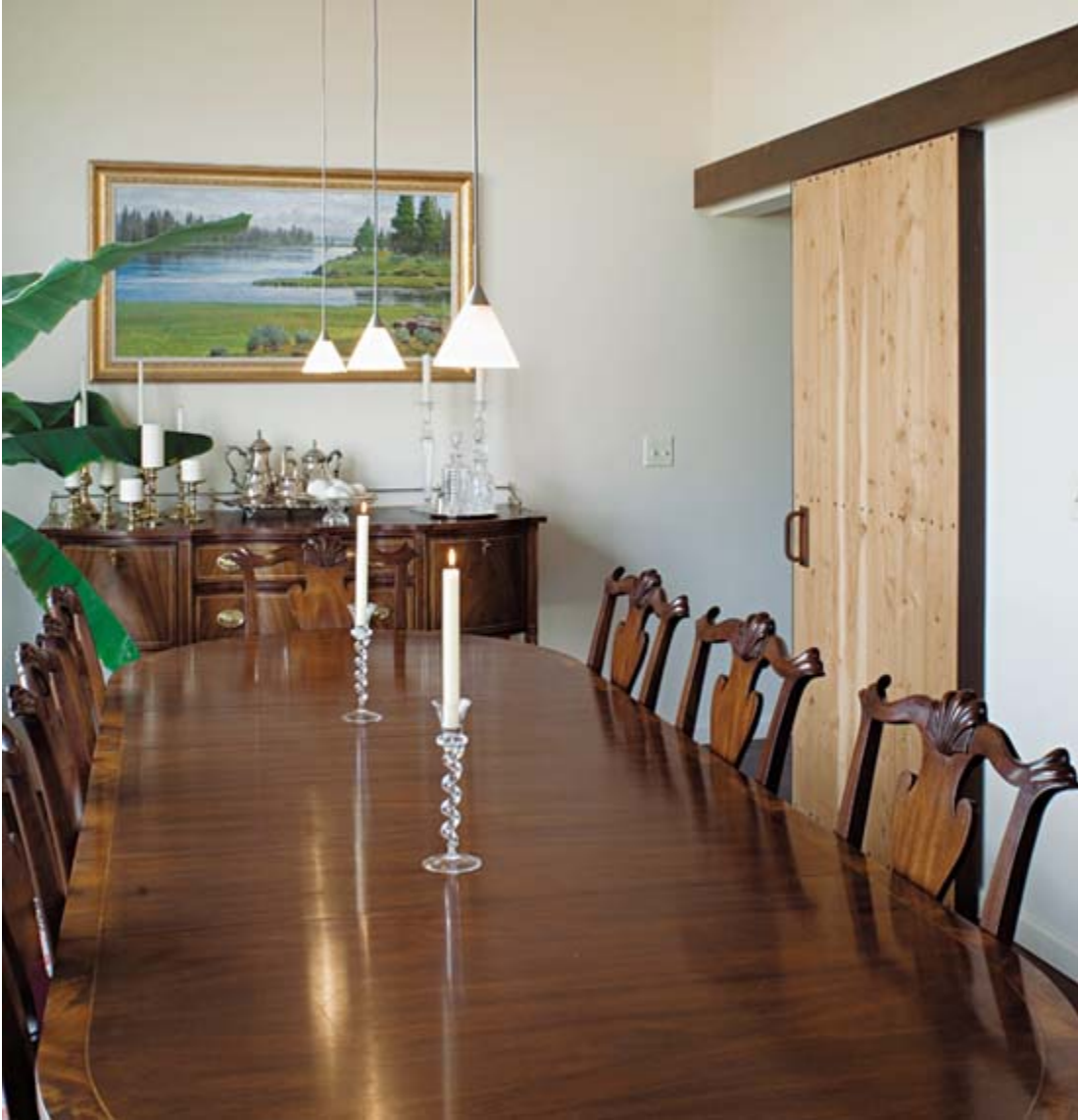
Custom-made surface mounted sliding doors built of steel and reclaimed wood provide openness or privacy between the rooms.
