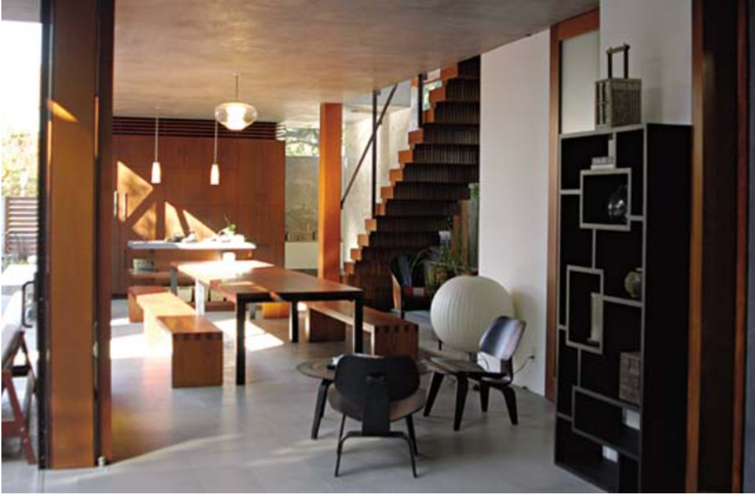
Concrete floors, with up to 40 percent fly ash in the mix, provide a sustainable and low-maintenance solution inside and out.
