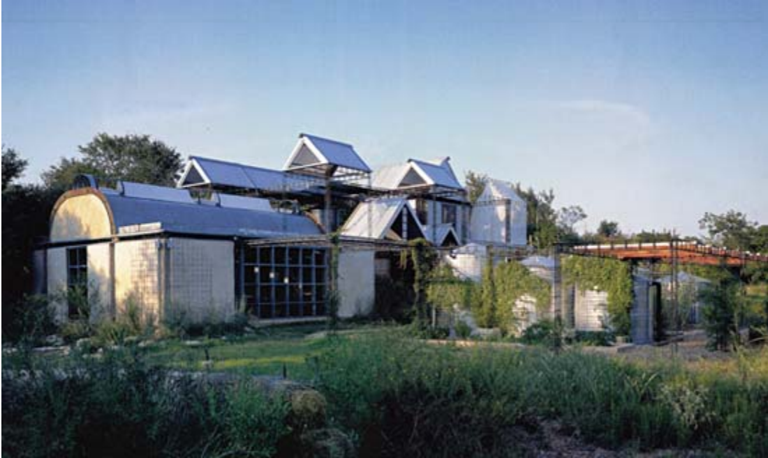
The center, with its vibrant collage of materials and forms is a direct expression of the variety of wall assemblies being studied.
