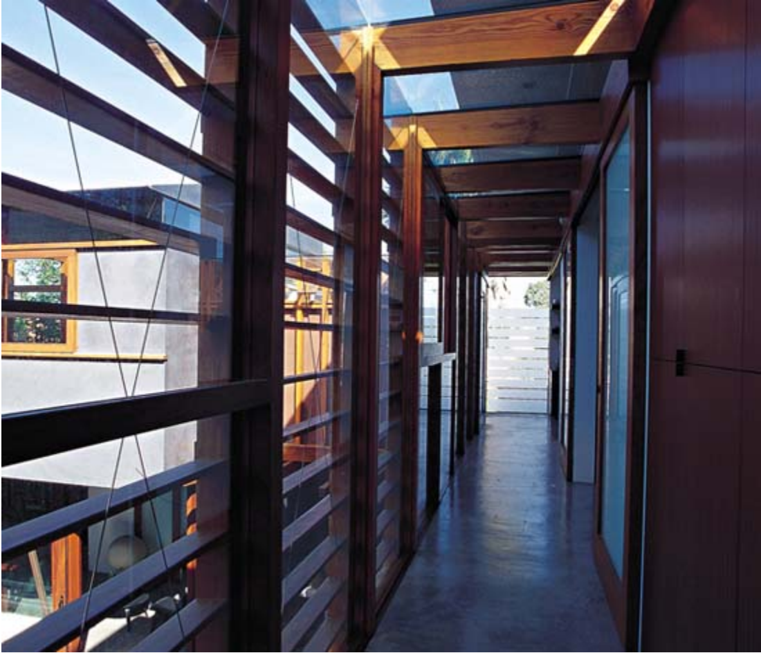
Louvers over windows at the second floor bridges provide a sun screen for the interior spaces.
