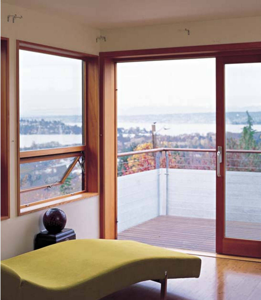
Large sliding doors open onto balconies built of Ipe, a FSC-certified lumber from South America, which has qualities similar to teak.
