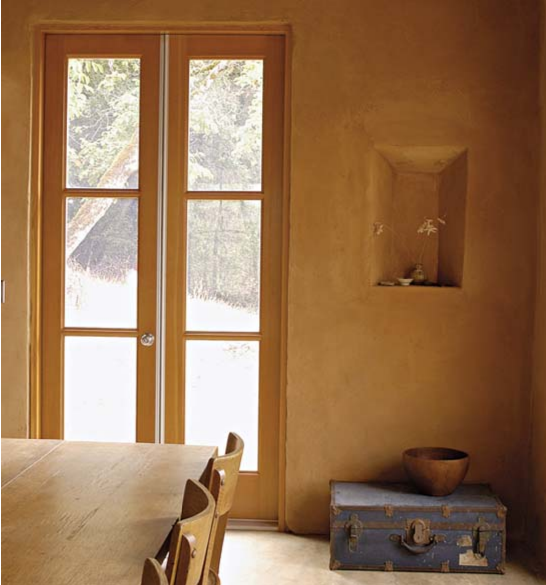
The thickness of the straw bale walls, finished with hand-troweled earth from the site, allows for niches to be built into the thickness of the wall.
