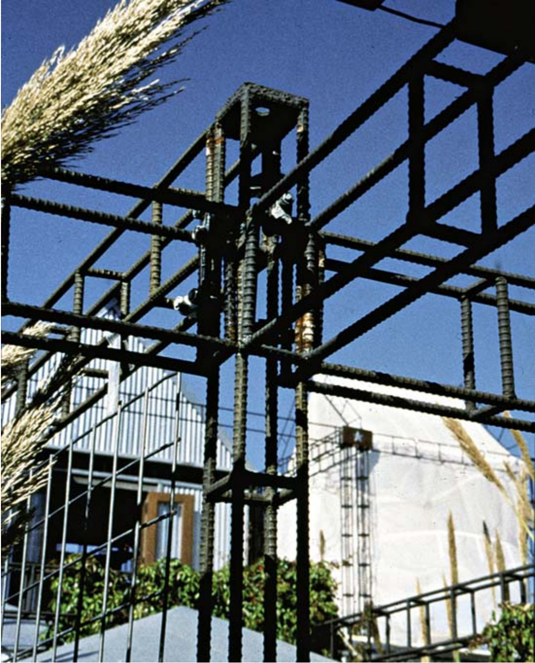
Fisk's GreenForms, built of steel rebar, provide a simple structural system on which to build.
