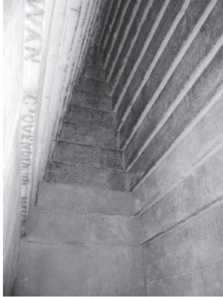
Figure 2.8. Corbeled ceiling in a chamber of the Red Pyramid. Courtesy of Jon Bodsworth.
