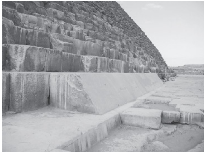
Figure 14.1. Original casing stones at the base of the northern face of the Great Pyramid. Courtesy of Jon Bodsworth.
